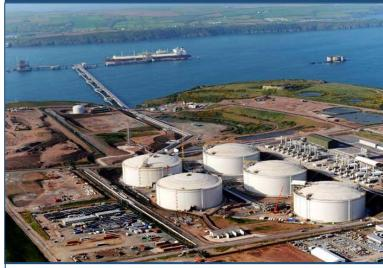
Upon arrival in the consuming country LNG is stored as a boiling liquid, which is then regasified for delivery to customers. LNG can also be used for peak-shaving and the growing market for SSLNG.
