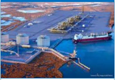
When gas fields are too remote from gas markets to be connected by high pressure pipeline, the gas can cooled to -161°C stored as a boiling liquid for transportation by ship and roadtanker.
